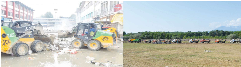
Figure 16: Fleet of trucks and JCBs to lift the waste
